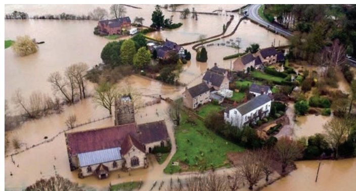
Severe flooding in Severn Stoke in February 2020
